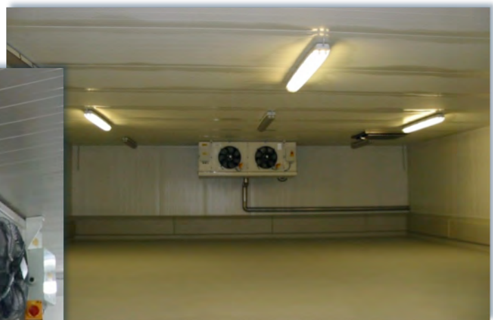
R404A evaporator in the cooling rooms
