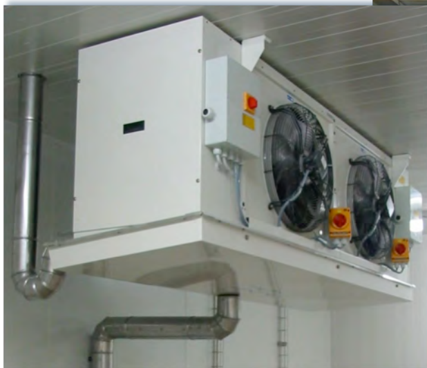
R404A evaporator in the cooling rooms
