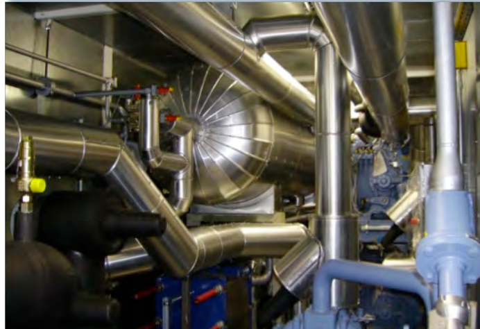
40 ft container with CO 2 / NH 3 soil-freezing containerised refrigeration system
